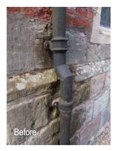
I am pleased to report that the church gutters and down pipes have been cleaned down, resealed and repainted using 2K primer and 2K polyurethane jet black paint, funded by our donation of £895.
